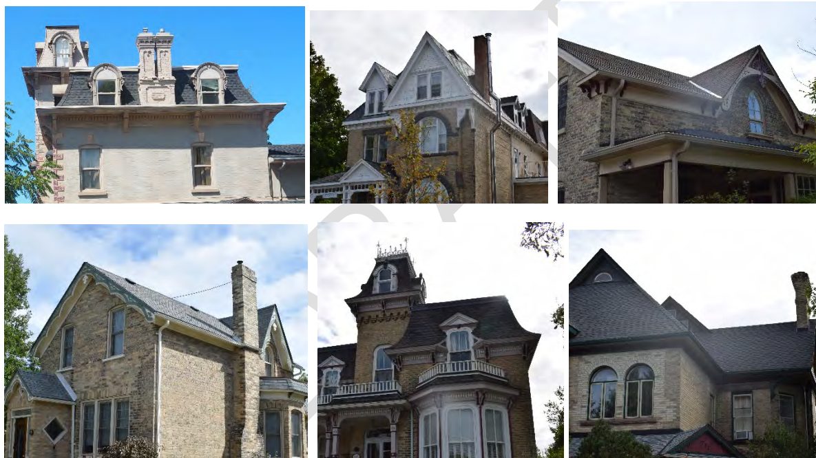
Plate 14: Examples of roof types in the Princes Street character area of the HCD. Most roof types consist of gables, mansard or hipped roofs, many with dormers and decorative woodwork at the cornices and pediments. Several of the gable and hip roof types maintain medium to steep pitch.
