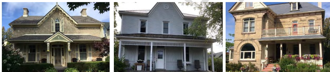
Plate 11: Examples of single-storey porches within the HCD. Typical construction includes wood post and beam, with decorative wood cornices, brackets, railings and spandrels.
