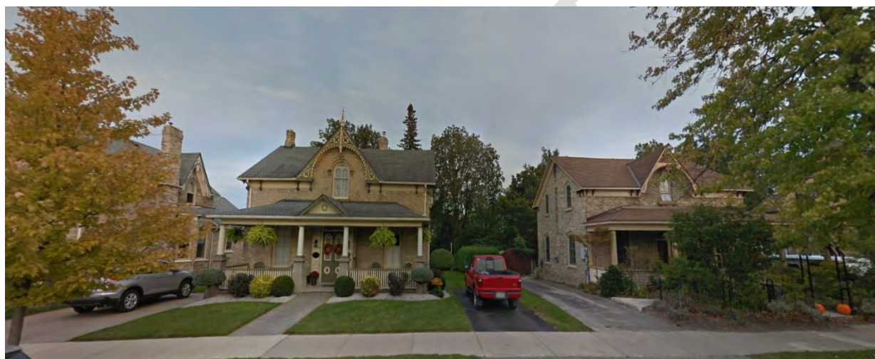
Plate 9: Maintain the datums created by single-storey front porch rooflines, one and one-half storey to two storey massing (as applicable), organization of fenestration along the first and second storeys, rhythm of two and three bays, use of buff brick as the primary façade material, and front-yard setbacks typical of traditional residential patterns in the HCD along Princes Street (Image Source: Google Streetview, 2020).
