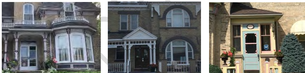
Plate 10: Examples of window and entrances located along Princes Street in the residential area of the HCD. Rectangular, round arch and segmental arch are most common. Many windows are 2/2 wood windows.
