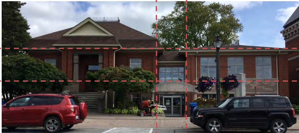
Plate 19: Example of the original Carnegie Public Library built between 1900-1920 in the HCD. The contemporary addition adjacent to the library creates a harmonious relationship between the heritage building and the new addition, through proportions, materials, and a separation between new and old.
