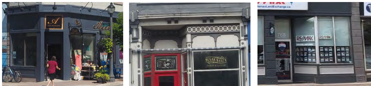
Plate 6: Examples of Wood in the HCD. Paneling, decorative detailing and pilasters are common.
