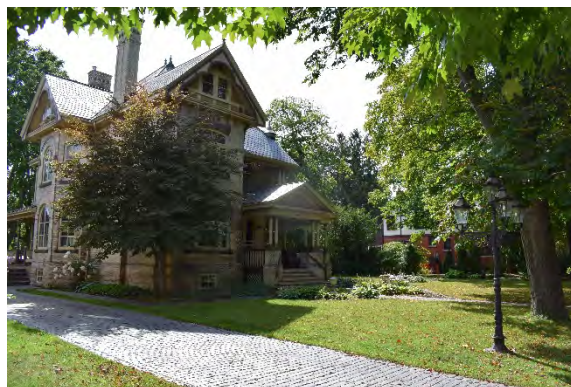
Plate 27: Driveways can consist of a variety of paving types, but should not be wider than one third of the lot, or 9 metres as limited in the zoning by-law
