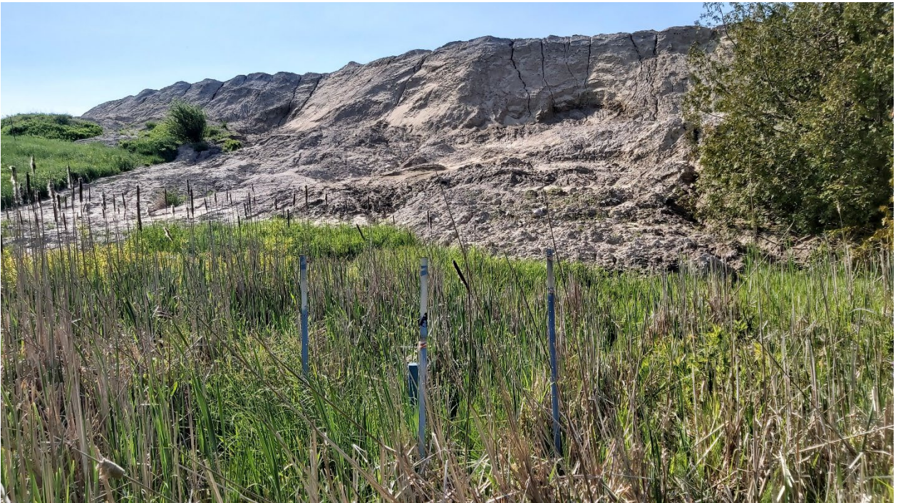
Photo 26 – West face of overburden stockpile on historic disposal area (Slope Inclinometer SI-03 in foreground) (May 31, 2022).
