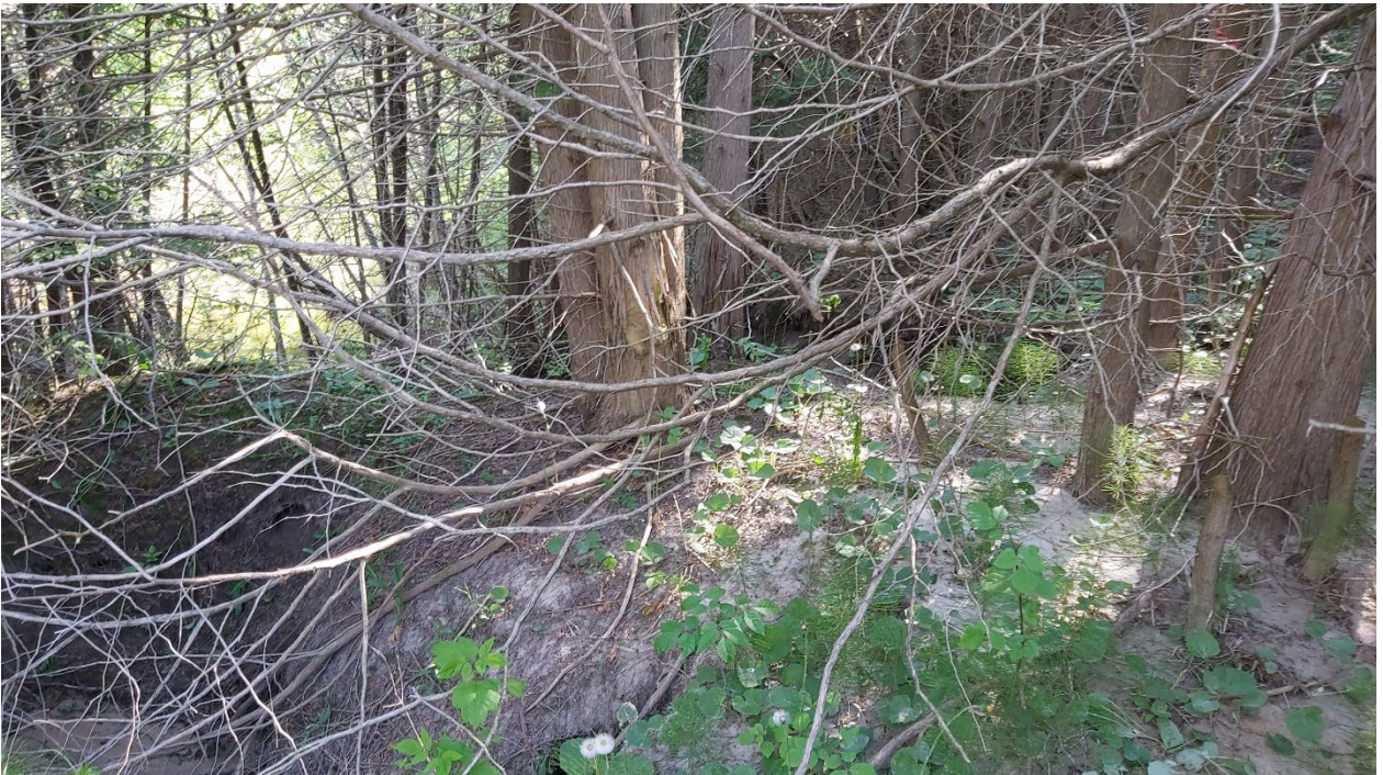
Photo 14 – Erosion gully north of Survey Pin SP-5, looking northwest (May 31, 2022)
