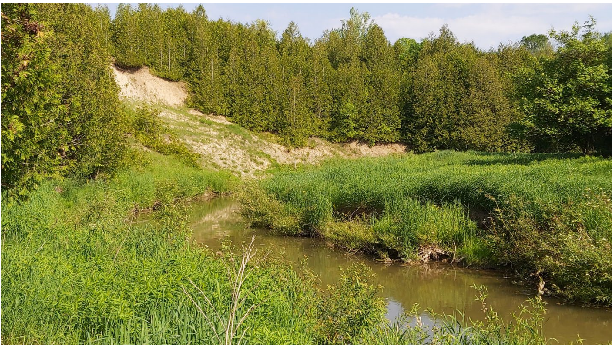
Photo 20 – Slope erosion near Survey Pin SP-6, looking west (May 31, 2022).
