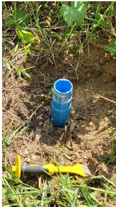
Photo 24 – Repair of Slope Inclinometer SI-01 in progress (May 31, 2022).
