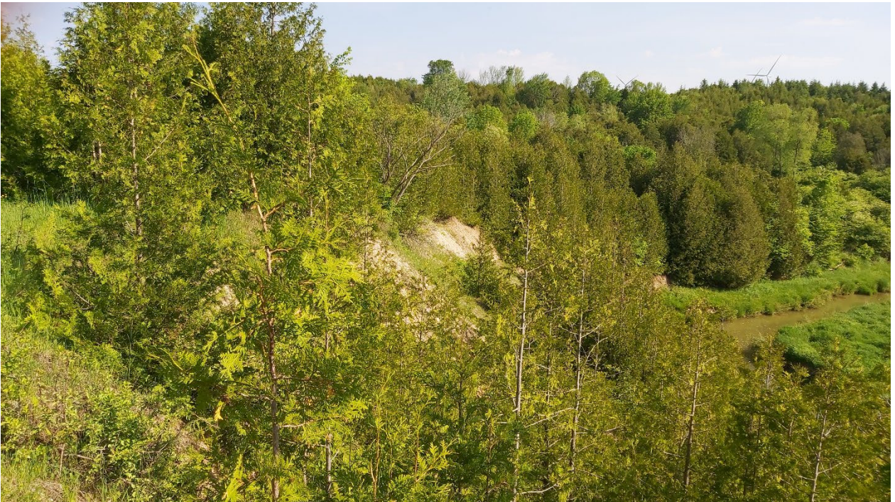
Photo 18 – Slope erosion near Survey Pin SP-6, looking northwest (May 31, 2022).
