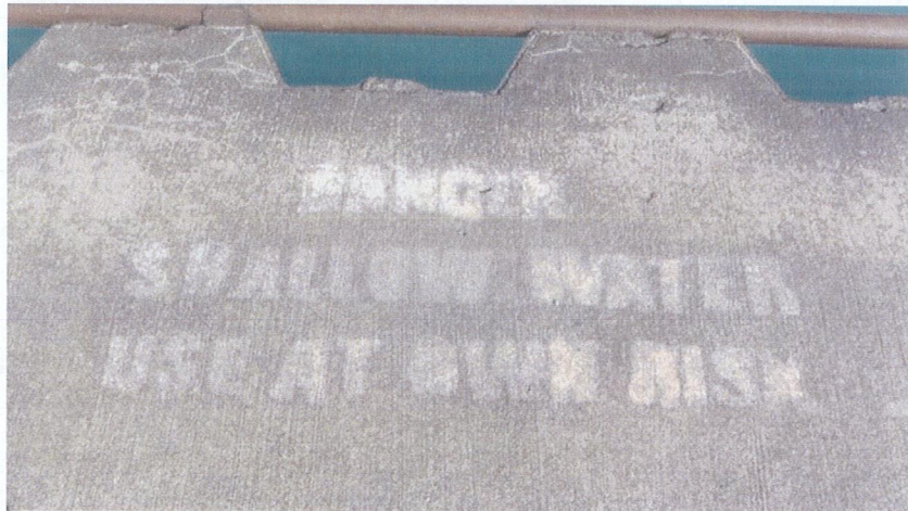
Existing signage on pier
