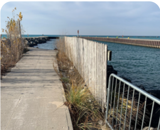
Entrance to South Pier. Access does not permit emergency vehicles to access.
