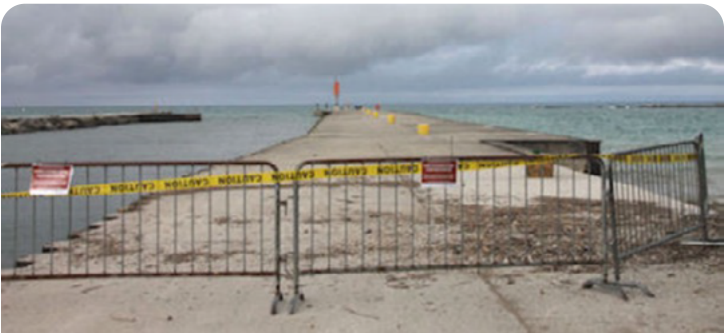
North Pier closed September 2023.
