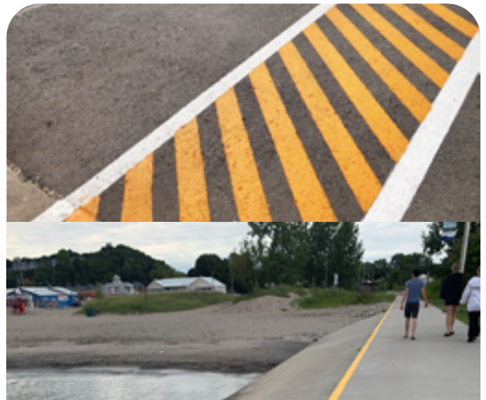
Example of painting to be considered on piers.
