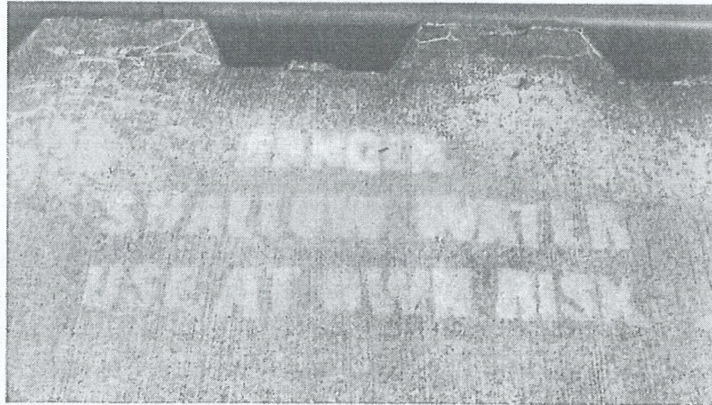
Existing signage on pier
