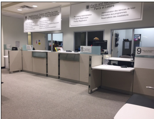
Example of service area and accessible service counter, Neighborhood, Children and Fire Services Office, City of London.
