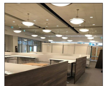
Example of suitable lighting level in City of London office environment with working and flooring surfaces that minimize reflective glare.
