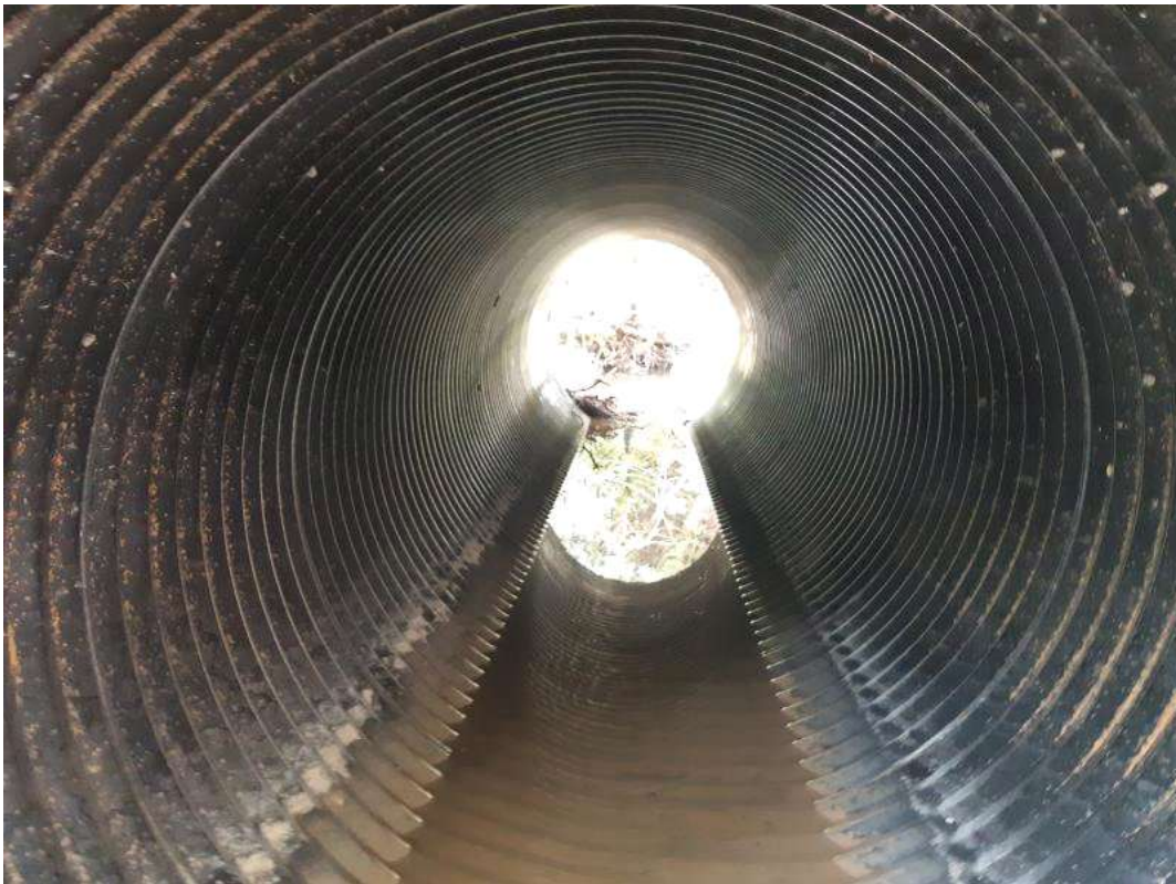
2-South Barrel Facing East
