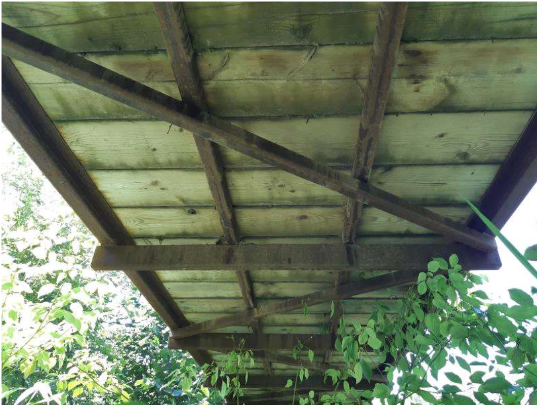
3-Soffit - North Span
